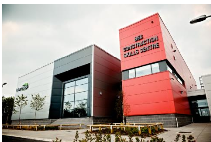
The £7m BEC Construction Skills Centre
