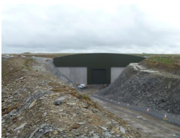
New vaults have been constructed at the LLW facility at Dounreay
