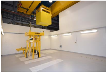
The estate's first Interim Storage Facility at Bradwell
