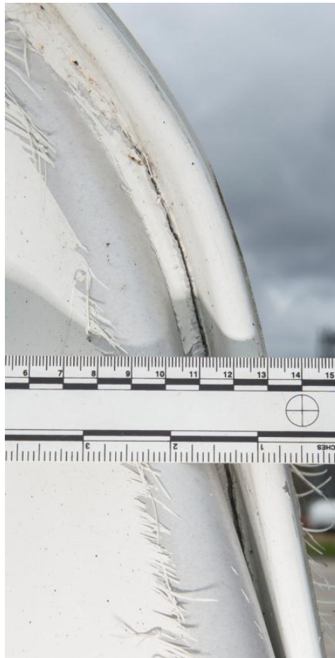
Figure 12. The 2008 tanker – rupture in the weld at top of impact zone
