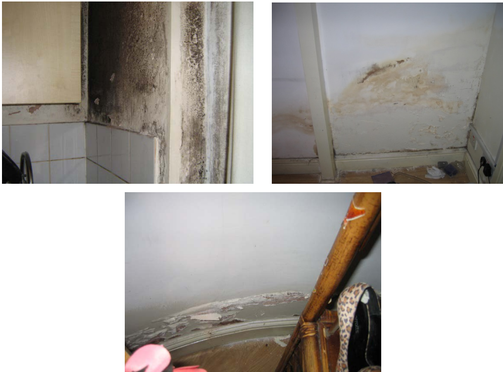
Figure 3.6: Homes with different types of damp
