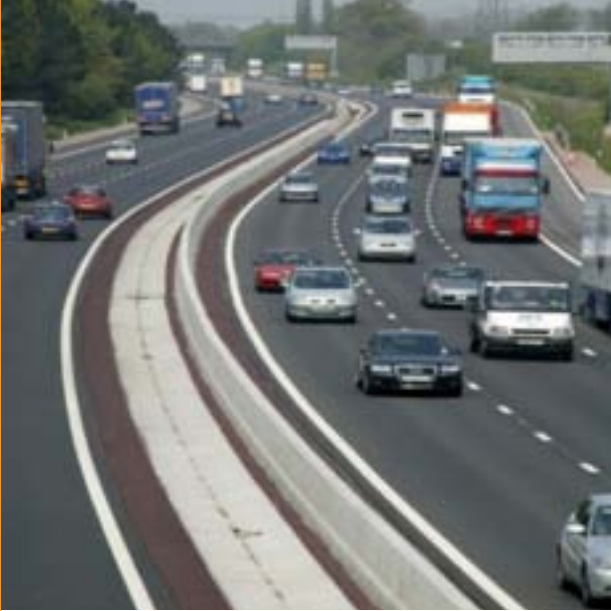
Figure 8: Concrete barrier in central reserve
