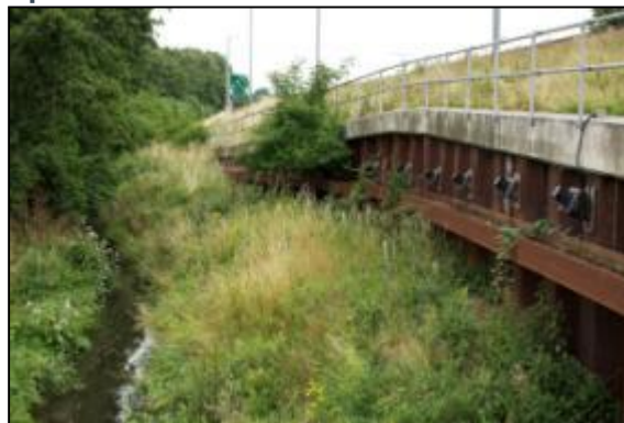
Figure 5-11 – Open Area on the Southern Bank of the River Ingrebourne
