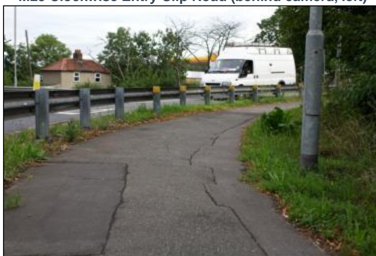
Figure 5-15 – Evidence of historic works to the Brook Street footway adjacent to the M25 Clockwise Entry-Slip Road (behind camera, left)
