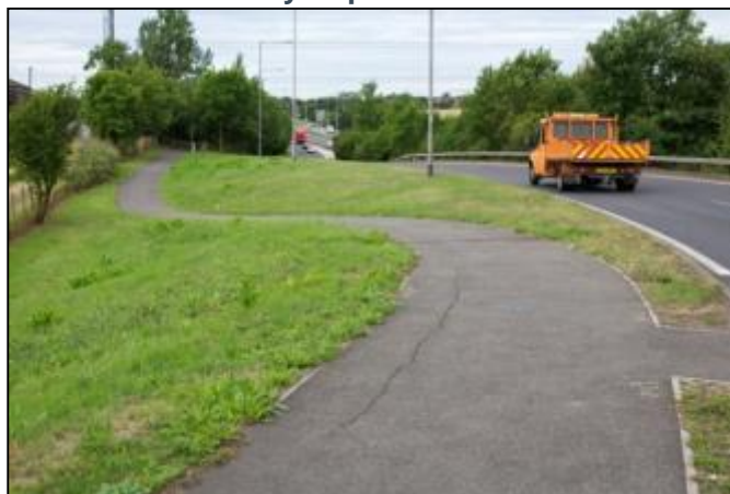
Figure 5-4 – Well Established Grassland Plots Performing Landscape Integration Function on the A12 Westbound Entry-Slip Road
