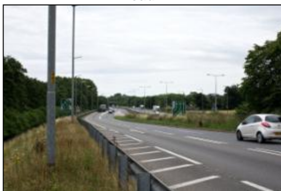
Figure 5-12 – Bat Deterrent Grassland Separating Linear Belt of Trees and Shrubs (used by Bats for Commuting and Foraging, left) and the A12 Eastbound Entry-Slip Road
