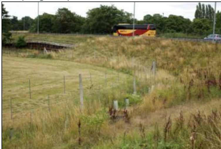
Figure 5-8 – Overview of Boundary Fence Planting the between the M25 Clockwise Exit-Slip Road (foreground) and the Extended Culvert and Retaining Wall (left)
