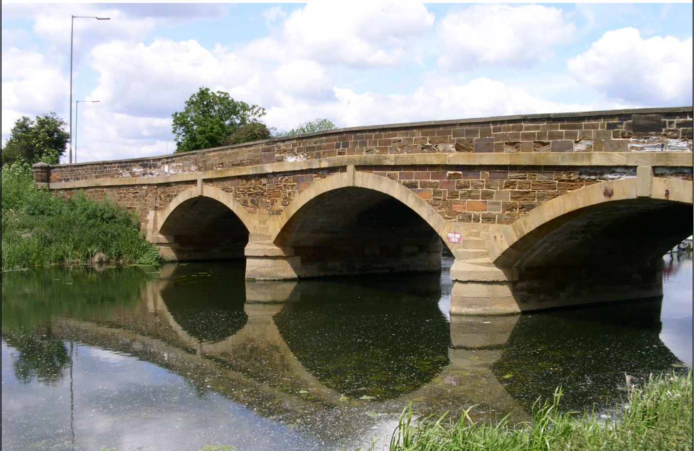
A1 Tempsford Bridge, River Great Ouse, Bedfordshire, Scheduled Monument and Trunk Road
