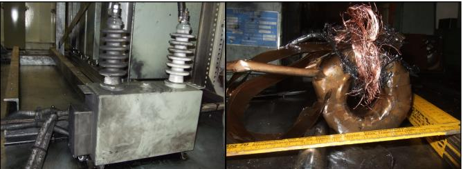
The current transformer used in imbalance current detection system
