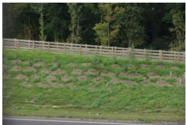
Poorly growing landscape planting on west side of the scheme north of Slacks Lane footbridge
