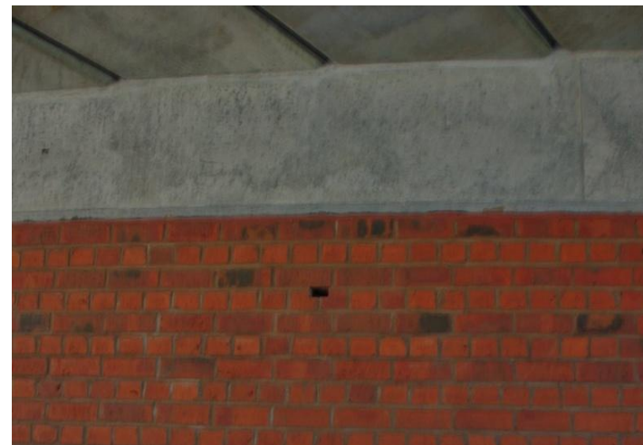
Figure G.4 – Bat roosts provided in new Grantham Canal bridge
