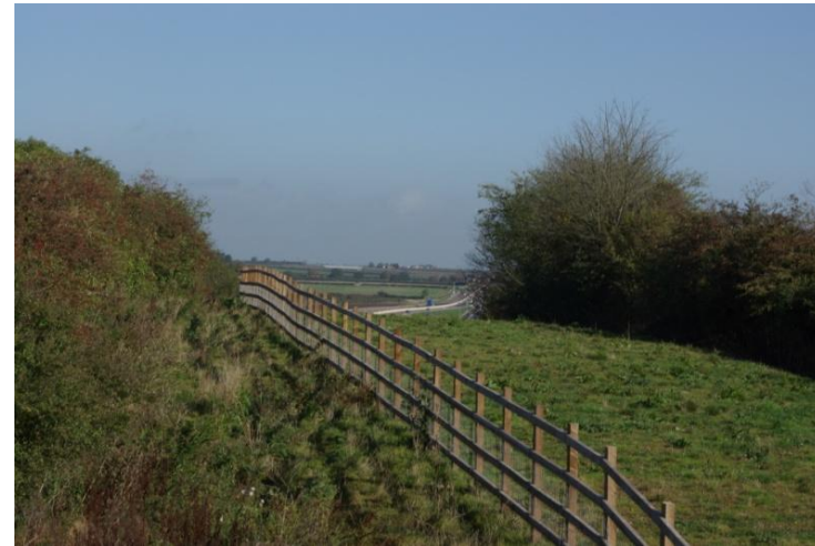
Figure G.2 – Retained SINC vegetation and seeded former A46 Cotgrave overbridge
