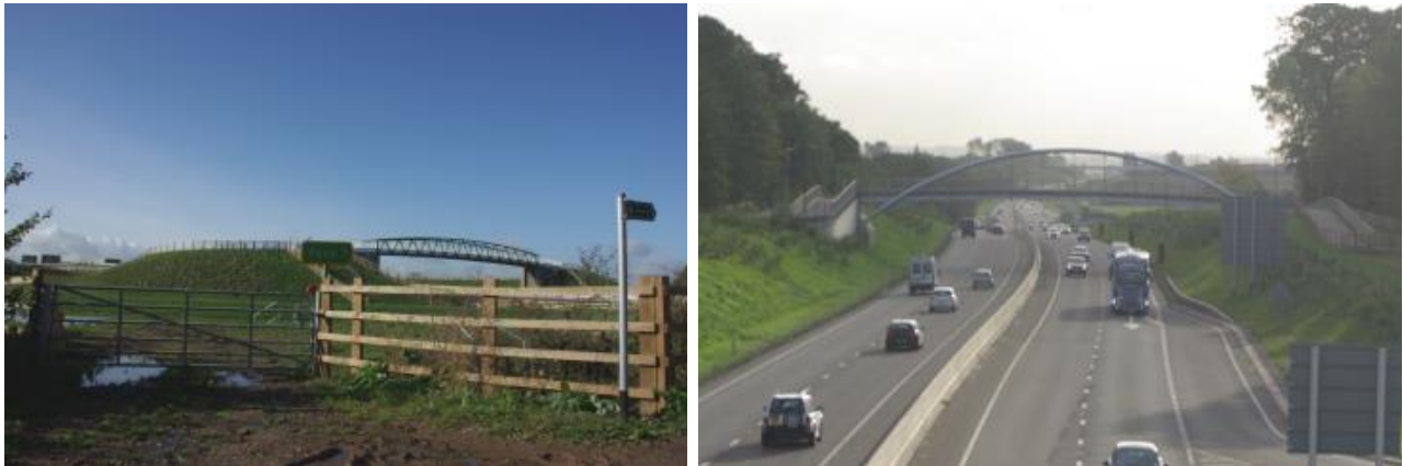
Figure 5-8 – Overbridges – Saxondale Bridleway viewed from the old A46 (left) and Slacks Lane footbridge viewed from Flintham Junction (right)
