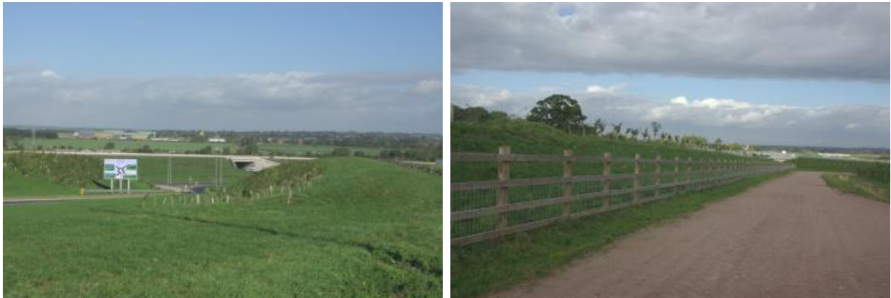
Figure 5-2 – Visual bunding at Saxondale (left) and view towards Syerston overbridge from Greengate Place (right)
