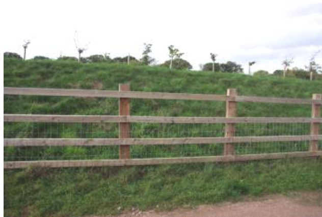
Figure 5-15 –Example of badger fencing south of Syerston overbridge
