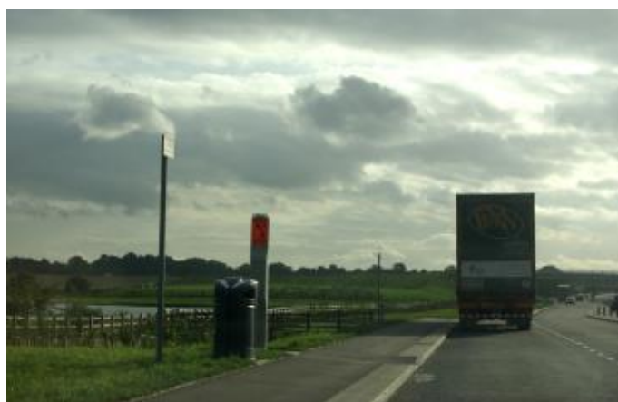
Figure 5-22 – Southbound lay-by north of Moor Lane over bridge
