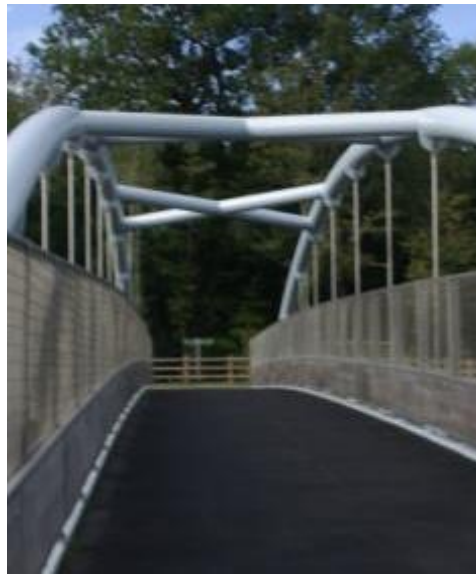
Figure 5-18 – Looking across Slacks Lane footbridge, showing high friction surfacing
