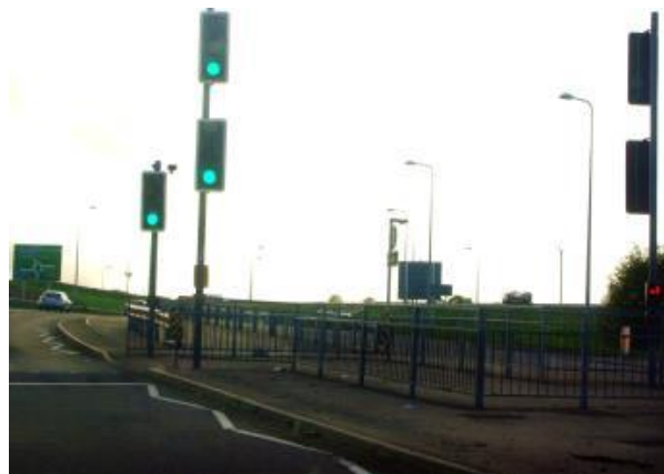
Figure 5-19 – New signalised pedestrian crossing on the A52 link road near Bingham
