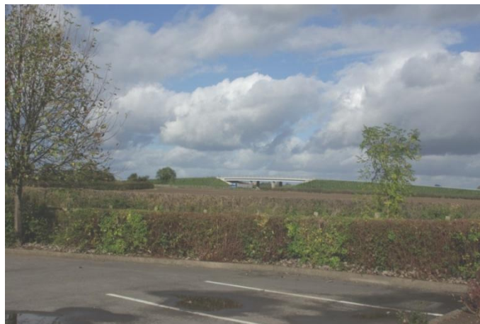
Figure F-4- Looking towards Butt Lane overbridge from car park of Bridgford Garden Centre (ST-79C)
