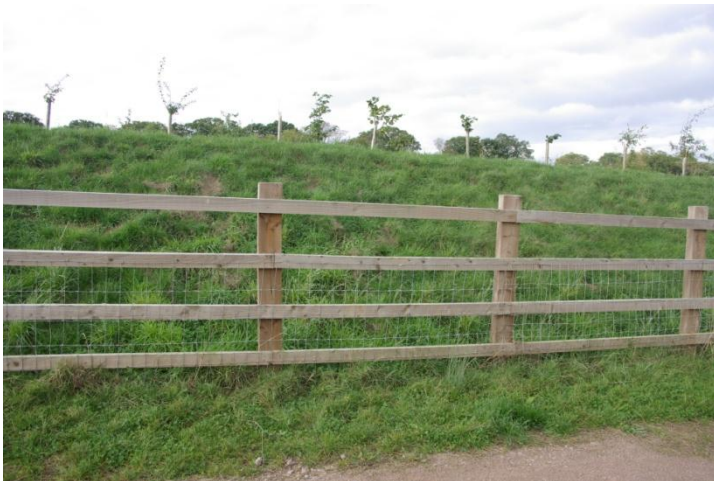
Figure G.7 – Badger fencing near Greengate Place
