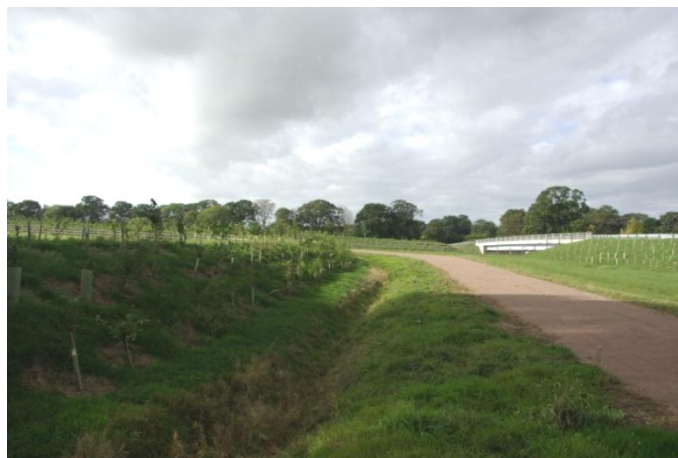
Figure F-5- View of the scheme seen by vehicle travellers on Greengate Place
