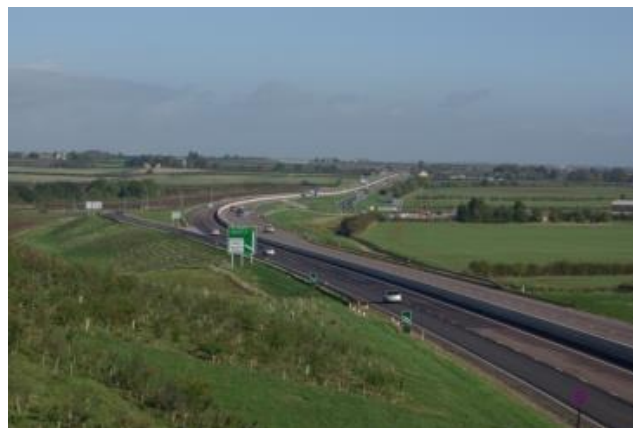
Figure 5-5 – Looking north from Cotgrave overbridge, with more established landscape planting in the foreground and less established in the middleground
