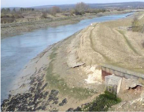
Plate 7 – Example embankment frontage requiring scour protection Reach 6
