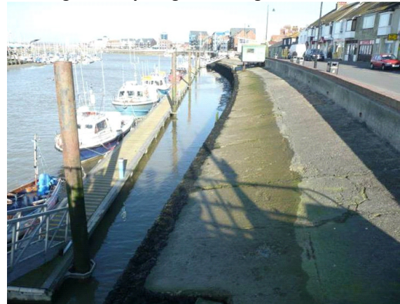
Plate 2 – Example Frontage Reach 2 (high tide) showing area requiring backfilling
