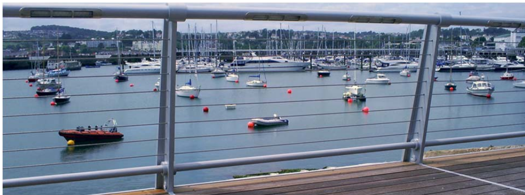
Image: Marshalls Torbay post and tension wire system, Torquay (Design by LDA Design)
