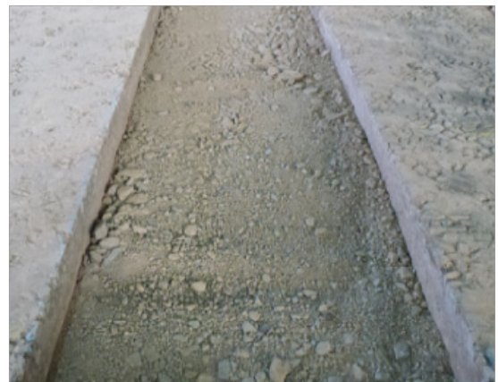
Figure 1 - Temporarily backfilled excavation
