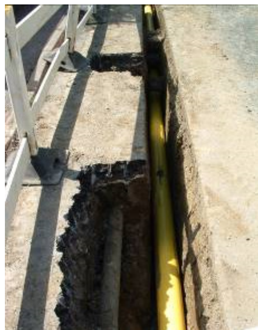
Figure 2 - Excavation where road plates are impracticable
