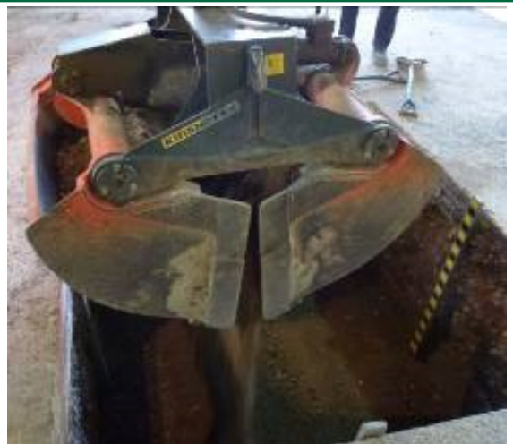
Figure 5 - Clamshell bucket depositing temporary backfill
