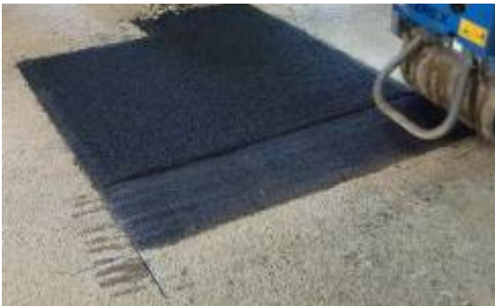
Figure 8 - Surcharge thickness applied to limit deformation
