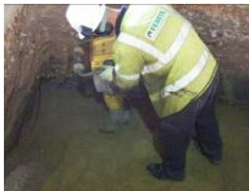
Figure 7 - Compaction of pea shingle during trials
