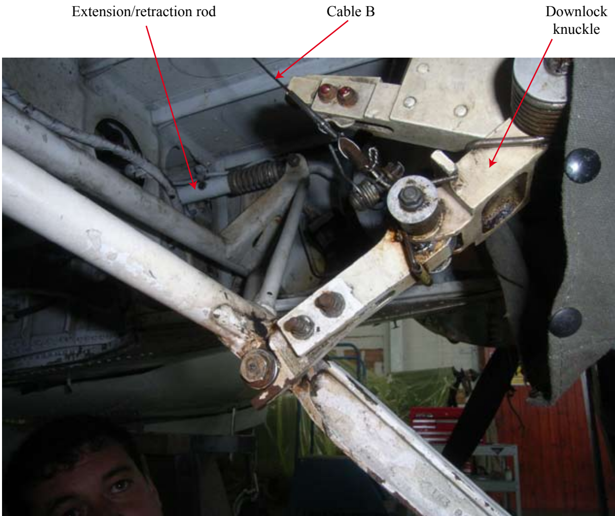
Figure 1 Gear down and locked
