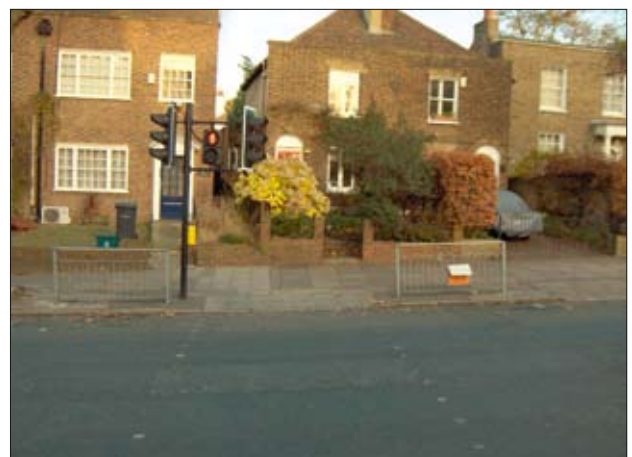
Fig. 3.6 Pedestrian crossing – were the guardrailings put in by default?
