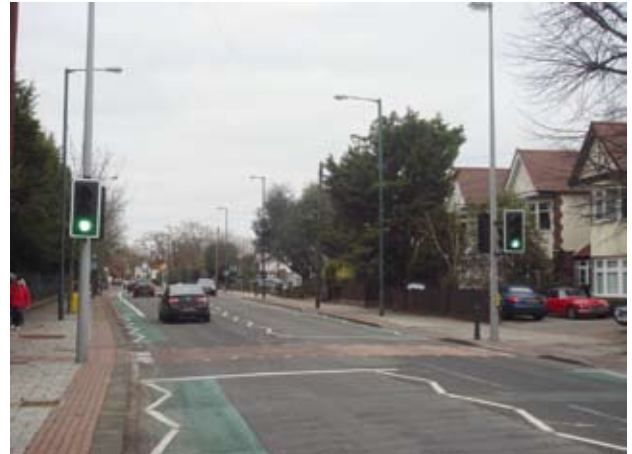
Fig. 3.4 A Pelican crossing where the signal heads have been mounted onto street lighting columns.
