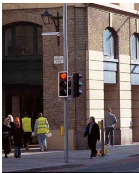
Fig. 3.1 Pelican crossing – signal heads mounted onto existing lamp column to reduce clutter, though a second push button mounting pole is provided, adding to street clutter.
