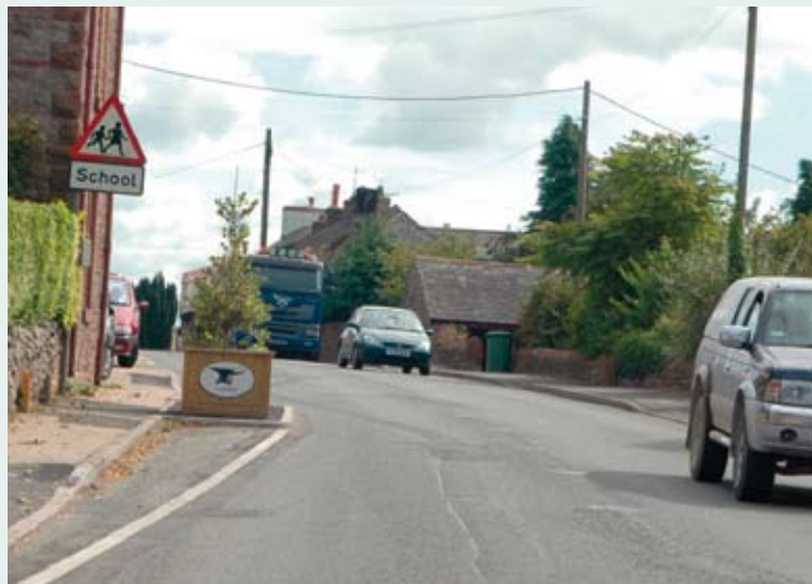
Fig. 5.2 A6 Clifton village after . Carriageway width reduced by kerb build-outs. The traffic calming effect is reinforced by the use of planters and by the removal of the road centrelines.
