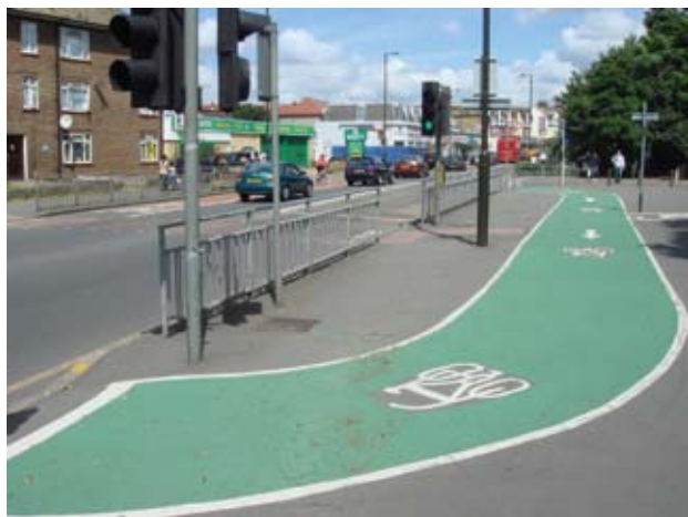
Fig. 2.1 Functionality acceptable, streetscape unacceptable.
