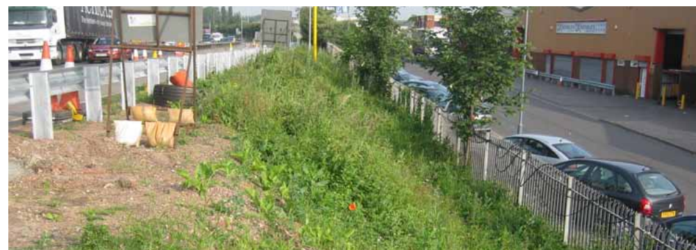
Slope no steeper than 1:2 with no hazards or obstructions
