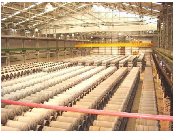
An Existing Store at Capenhurst
