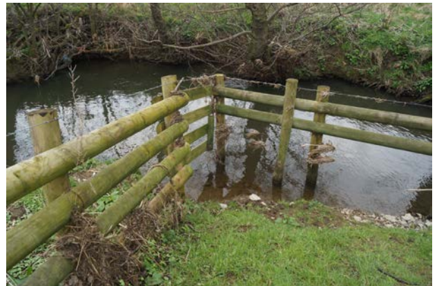
Cattle drinking point installed on River Ecclesbourne at Duffield
