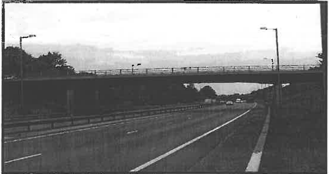
General view of structure, looking southbound
