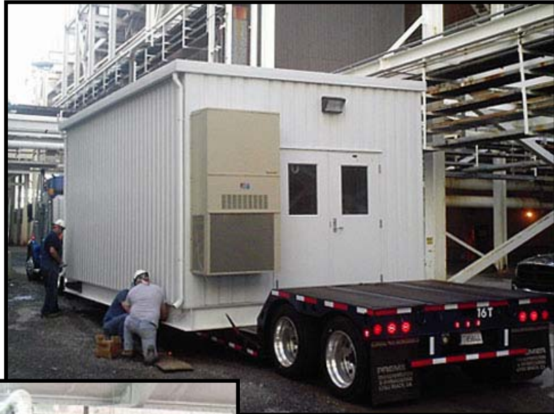
Modular Control Room
