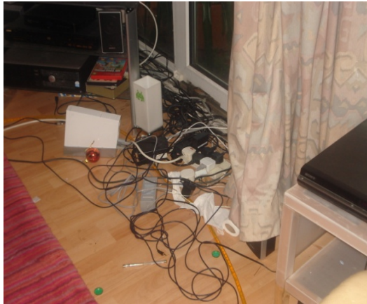
Figure 3.3: Examples of inadequate electrical safety that increase the risk of fire in homes
