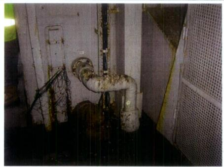
Material Comments: Isolated section of asbestos containing debris to pipework with non asbestos insulation. The debris to this pipework was of unknown origin.
