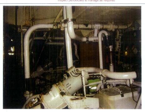
Material Comments: Asbestos containing gasket material sampled from pipework. Due to the extent of pipework throughout this area it is likely that a mixture of gasket materials will be present to flanges
