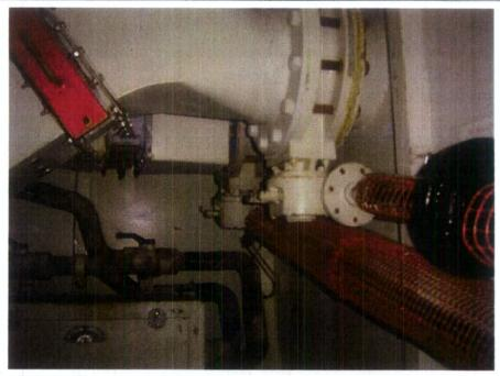
Material Comments: Asbestos containing gaskets to 2 No. cylindrical sections of ducting, which exit through wall.
