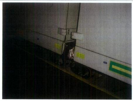
Material Comments: Asbestos containing woven textile conduits, as Loc Ref: 245, at low level between cabinets and to wall adjoining 909 annexe.
