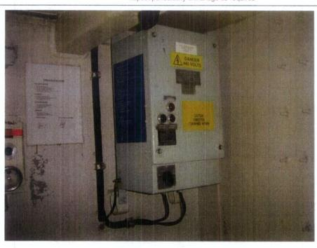
Material Comments: 1st space has foam and MMMF lagged pipework. Fuse box to wall with asbestos warning sticker applied. Presume asbestos cement guards, or asbestos fuse tape within.
