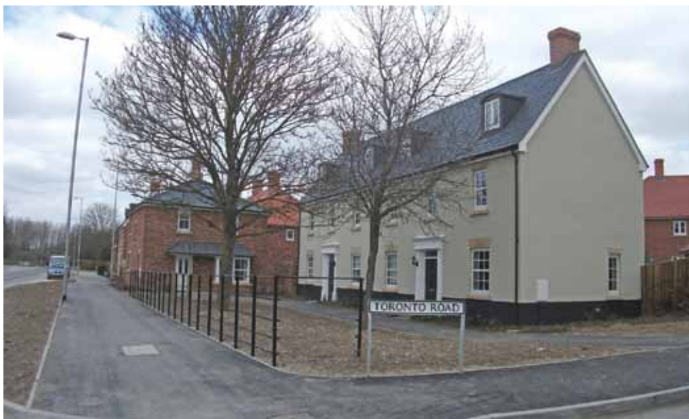
New Service Family Accommodation at Canada Lines in Bulford
