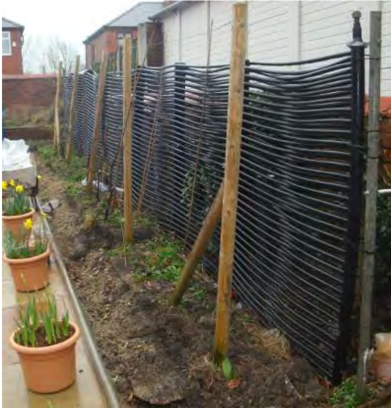
Figure 1 – Energy Fence hybrid ground and air heat collector
