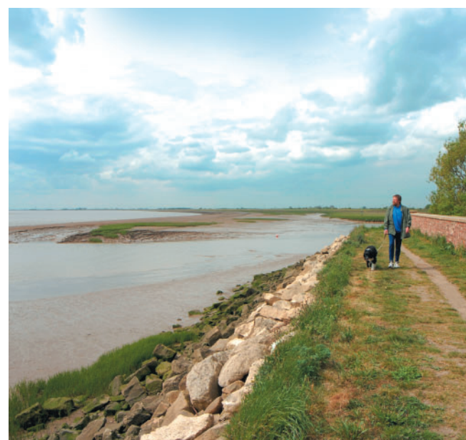
Flood defence at Brough
