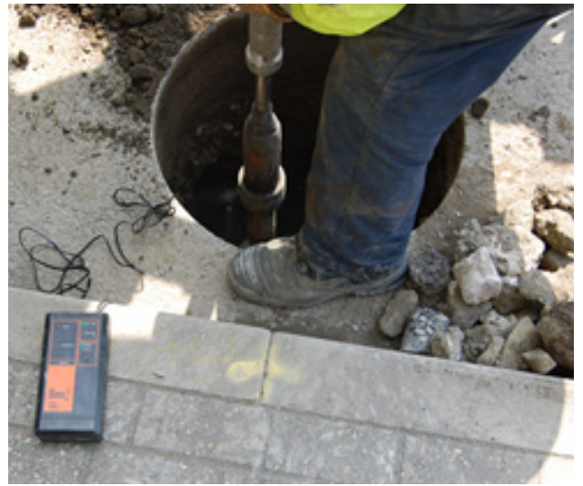
Figure 13 - Grouting the core back into place to match the original surface level and orientation
