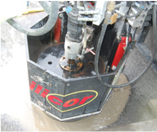
Figure 10 - Vacuuming out the exposed unbound material, after loosening where necessary
