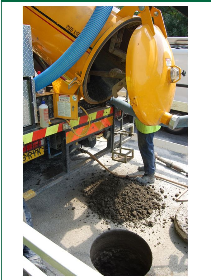
Figure 2 - Core and Vac in use
