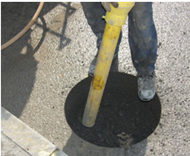
Figure 10 - Vacuuming out the exposed unbound material, after loosening where necessary
