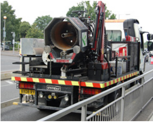
Figure 9 - Coring through the bound layers
