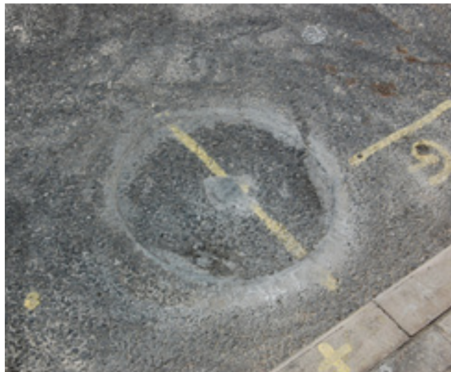
Figure 6 - Appearance of reinstatement on completion
