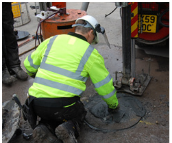
Figure 13 - Grouting the core back into place to match the original surface level and orientation
