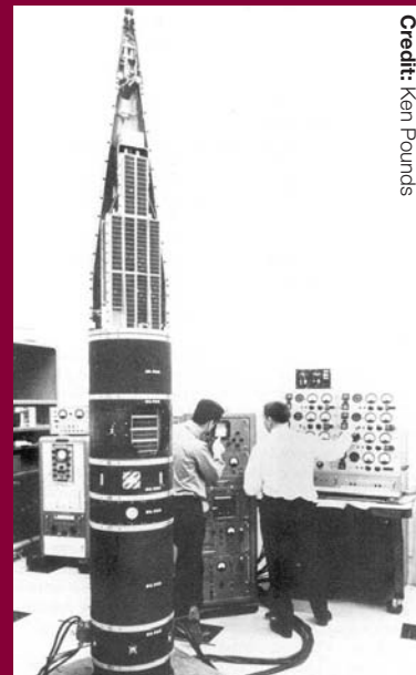
Tests being carried out prior to launch on an early Skylark payload at Woomera
