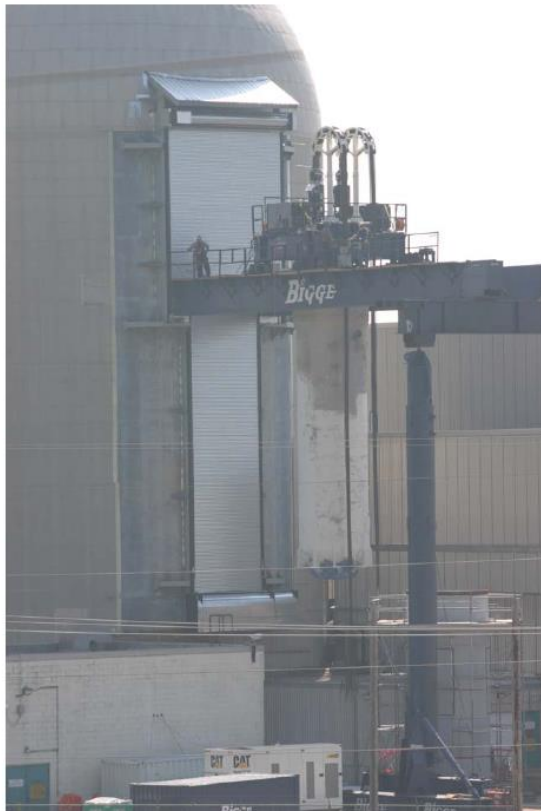
Removal of the Reactor Pressure Vessel (RPV) from the reactor building
