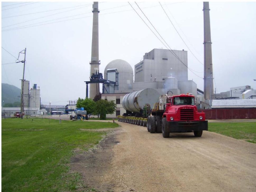
Transfer of the RPV transportation package to the rail siding
