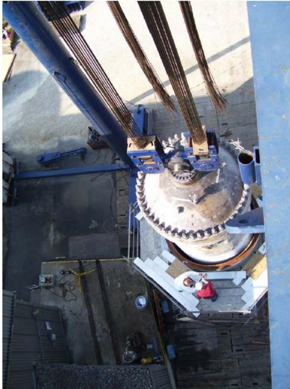
Set down of the RPV in the lower half of transportation canister
