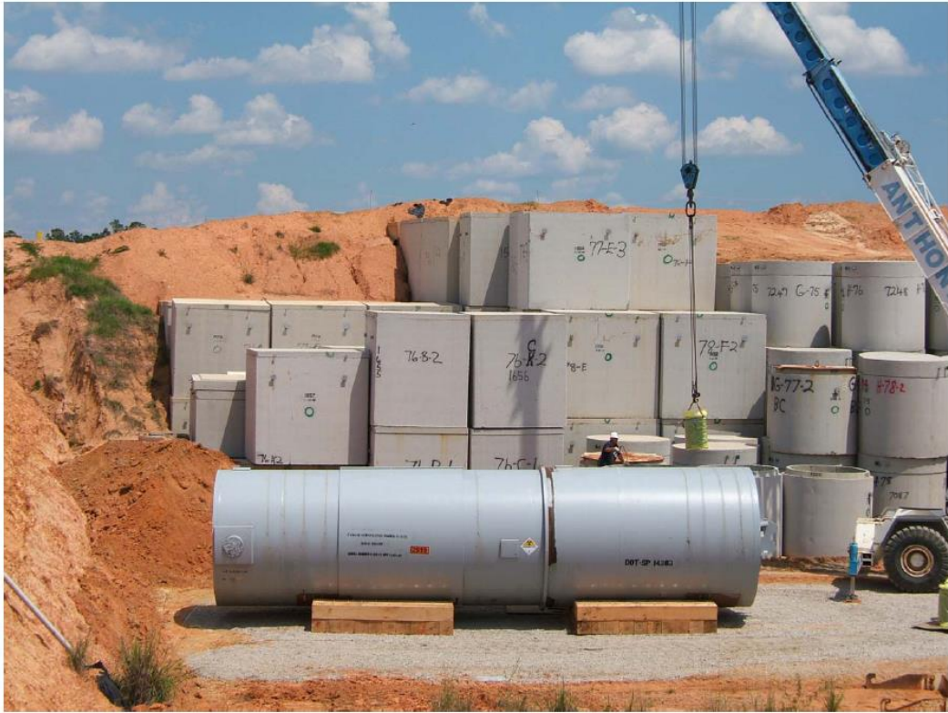
Final placement of RPV transportation package in disposal trench
