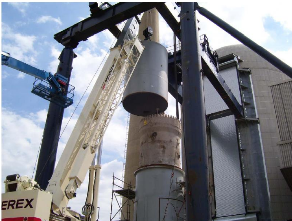
Set down of the RPV in the lower half of transportation canister
