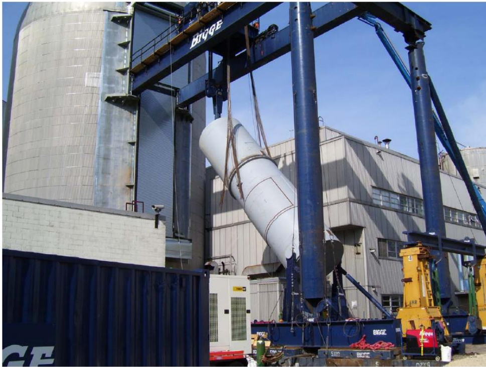
Downending of RPV transportation package for transfer
