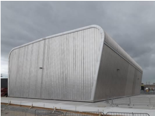
Bradwell ILW Store
