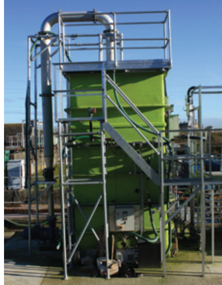
CCD aerator being tested
