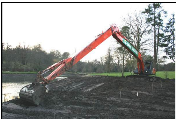
Plate 4: Large long-reach excavator.
