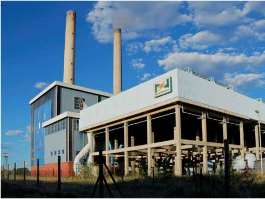
The Van Eck coal-fired power station in Windhoek
