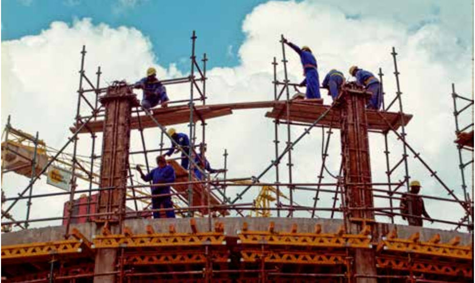
Construction workers busy working on site
