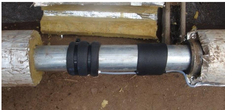
Figure B 13 – Temperature probe being mounted on a steel pipe.
