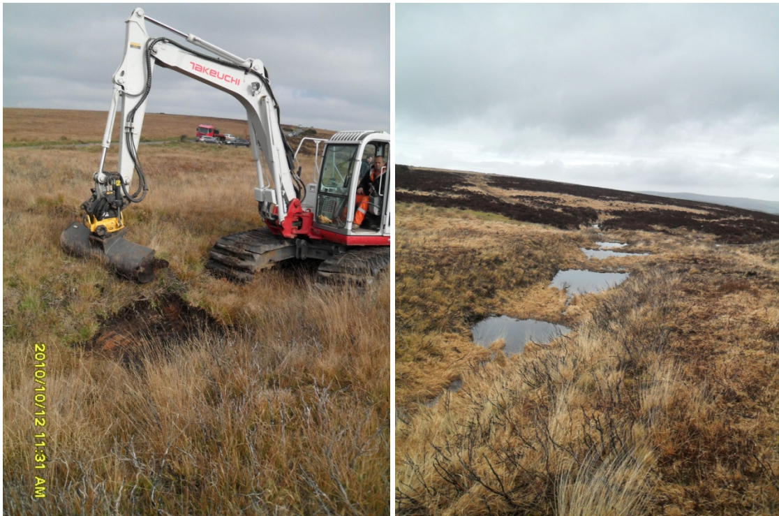
Figure 2.6 Upland ditch blocking undertaken by the National Trust in the upper reaches of the Horner Water catchment in October to November 2011 with the aim of increasing water storage and reducing the velocity and magnitude of discharge response to rainfall events
