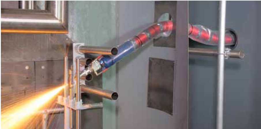
Cutting target pipes after cutting obstructing pipes within the vessel.
