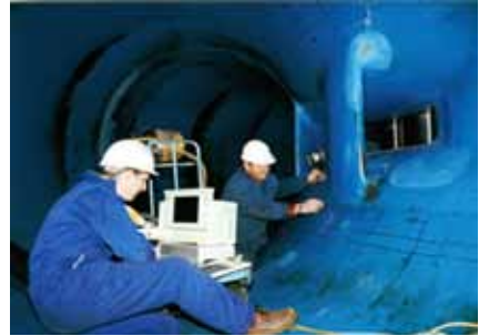
On site NDT inspection.
