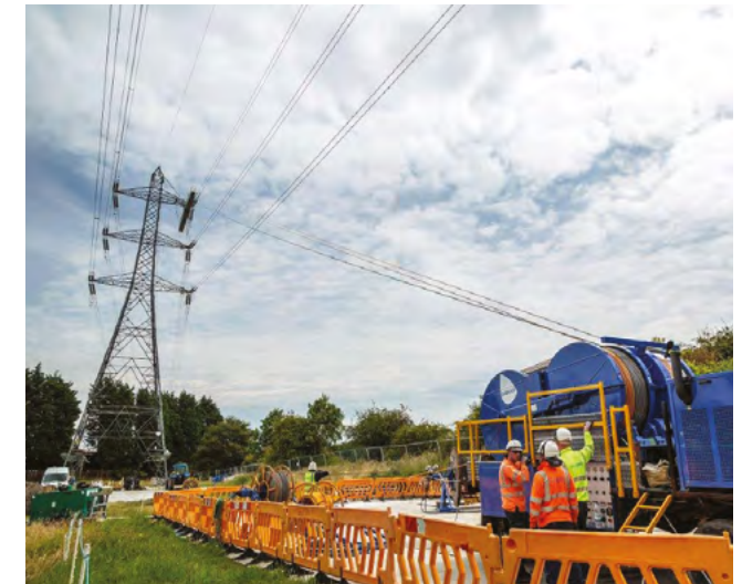
Typical winching site
