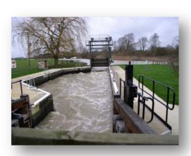
The photograph above shows how a lock may be used to discharge flood water on the River Great Ouse when Strong Stream Advice has been issued.
