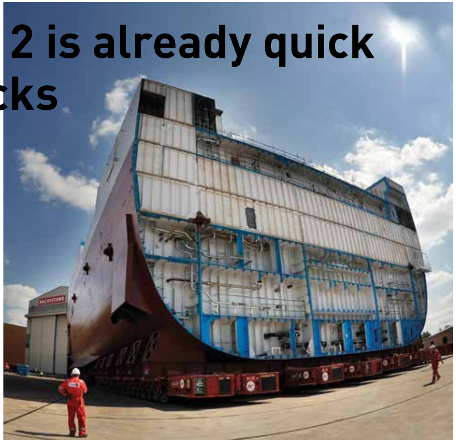
Round the block: Lower Block 03 of Queen Elizabeth , giving an idea of the sheer size of the carriers. Prince of Wales ' block is close to its journey to Rosyth
