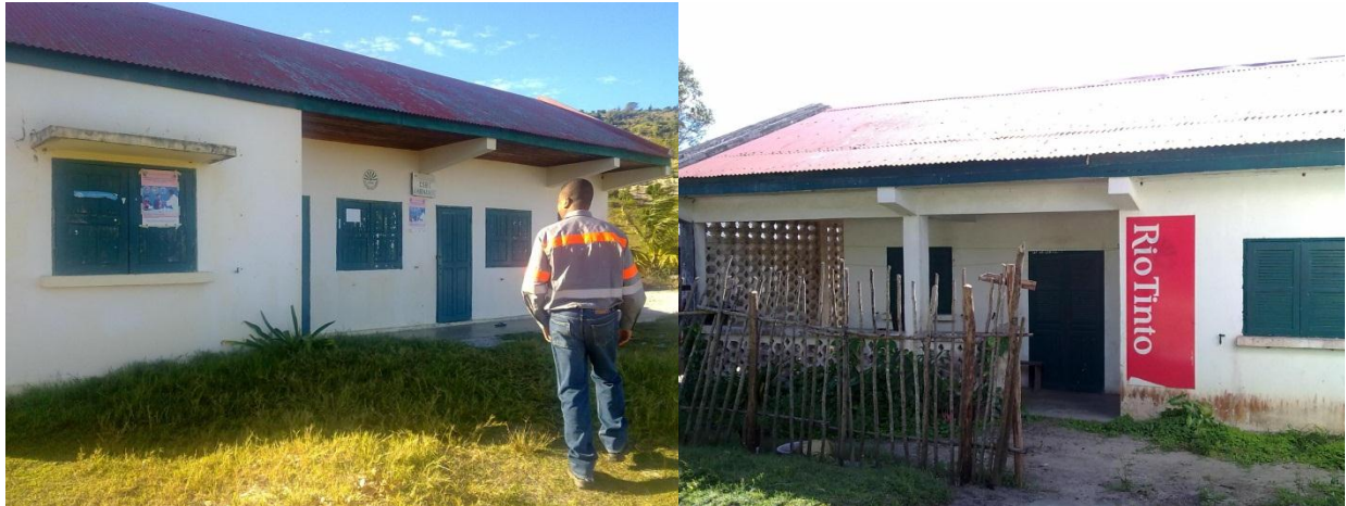
Figures 6 and 7: Health centre and staff accommodation built by RTQMM
