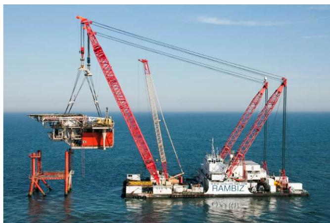
With the topside removed work platforms were established on the jacket to allow for the cutting and removal of the leg extensions and placement of the abrasive cutting tool into each of the legs for cutting. Each leg was cut at least 3m below the natural seabed. As each leg was cut a rigging arrangement was attached to the top of the jacket allowing the HLV to lift the jacket clear of the seabed immediately
