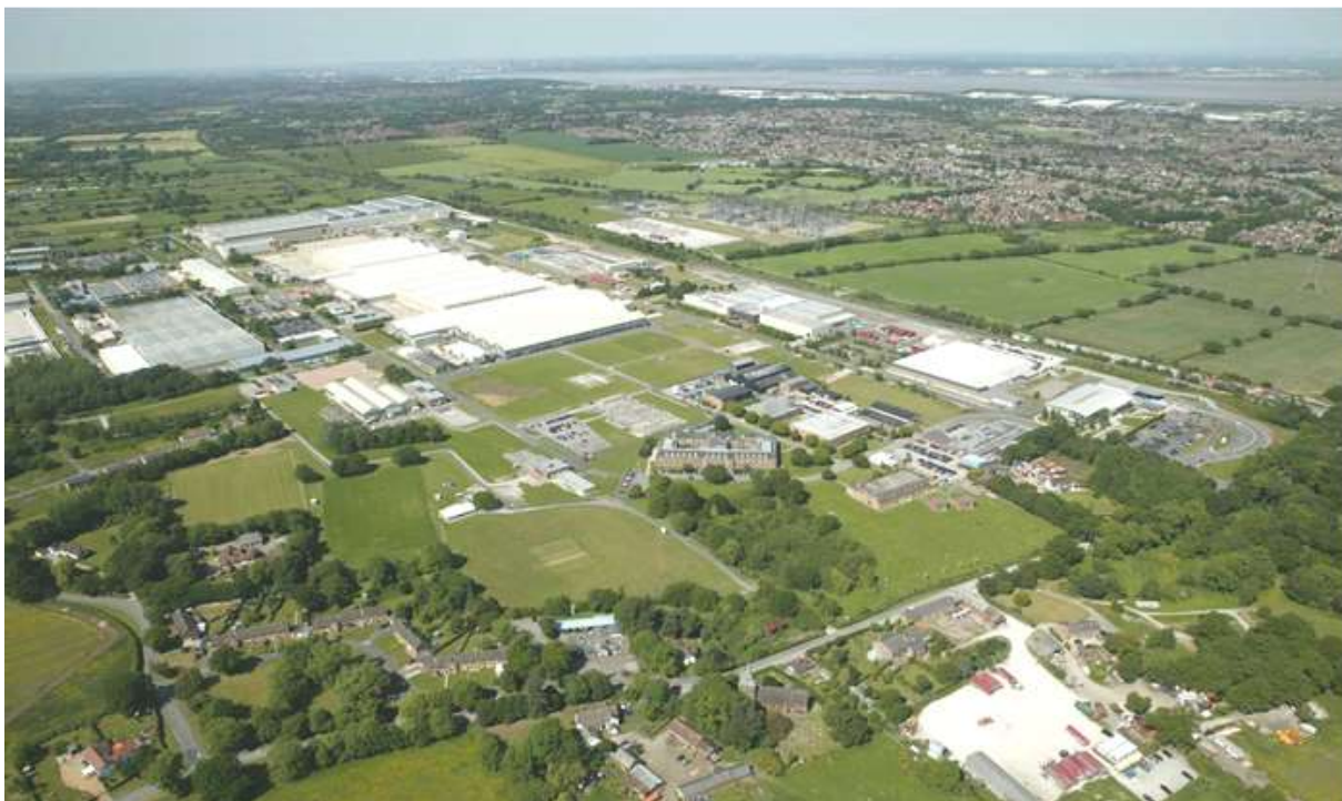
Figure 5-7: Aerial view of Capenhurst (CNS)
