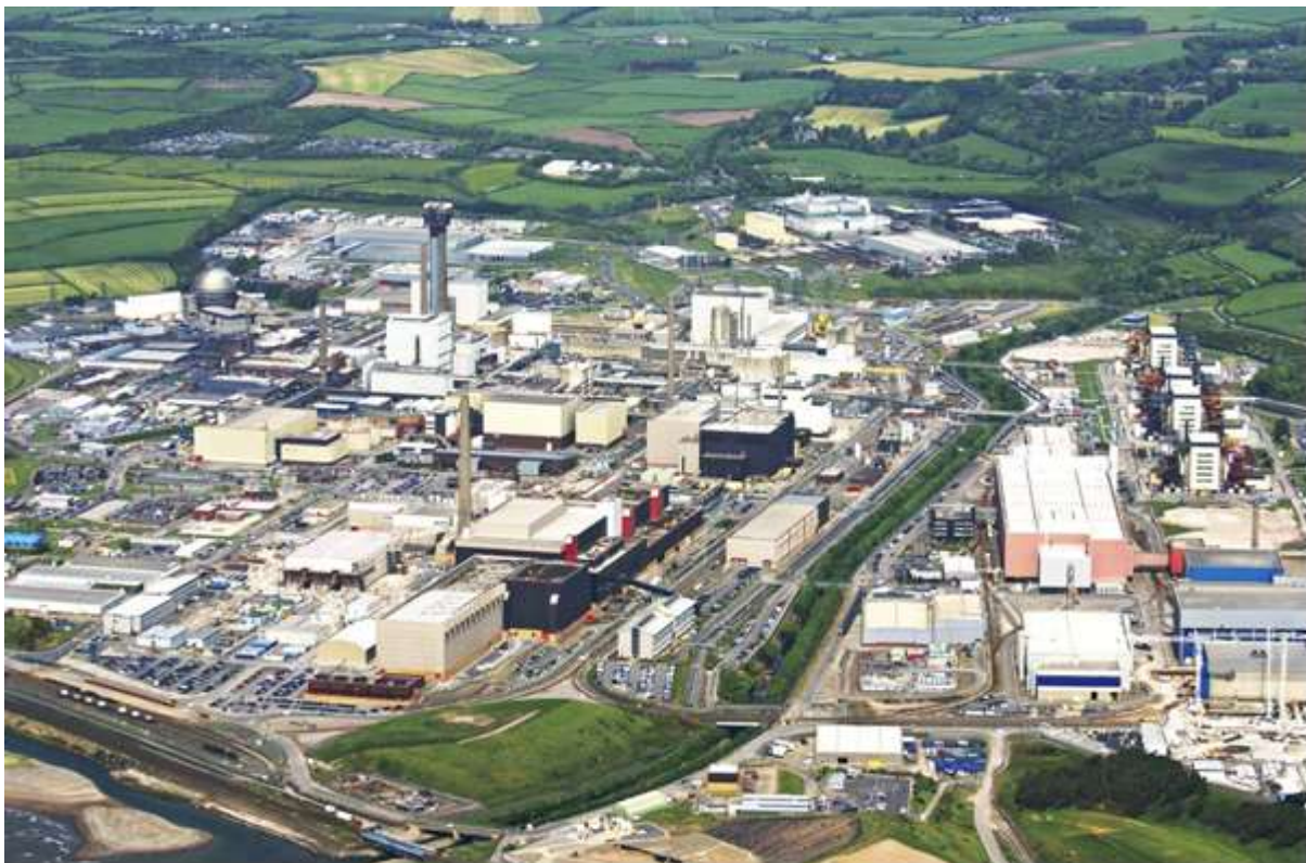
Figure 5-10: Aerial view of Sellafield
