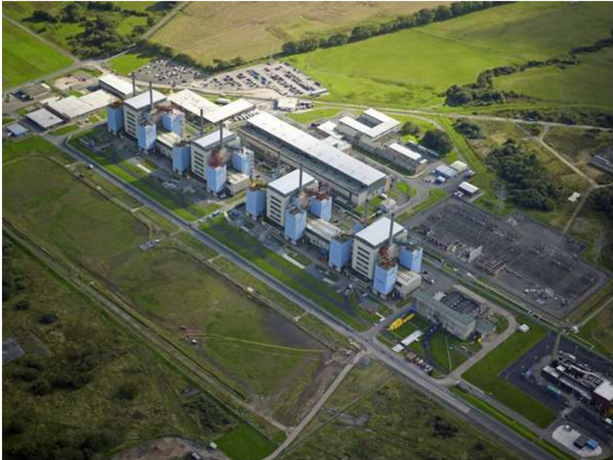
Figure 5-13: Aerial view of Chapelcross
