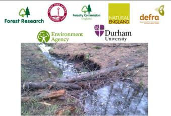
One of >150 large woody debris dams constructed in woodland streams to 'slow the flow'
