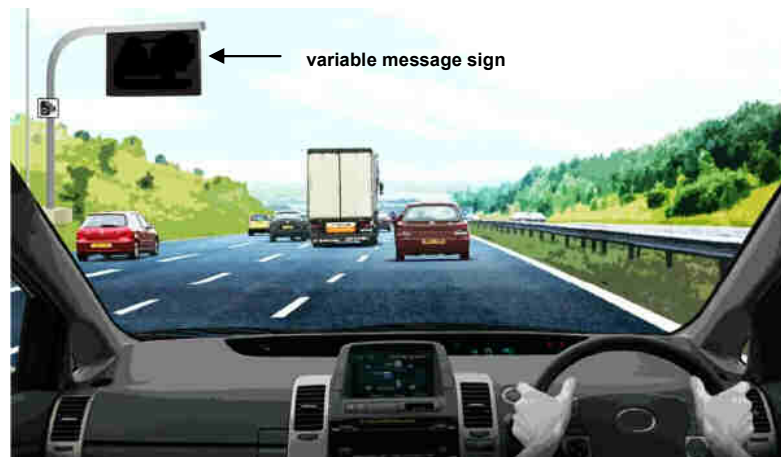
Figure 4B: Illustrative M1 J28 to J31 managed motorway scheme section operating in normal motorway conditions with a blank verge mounted variable message sign
