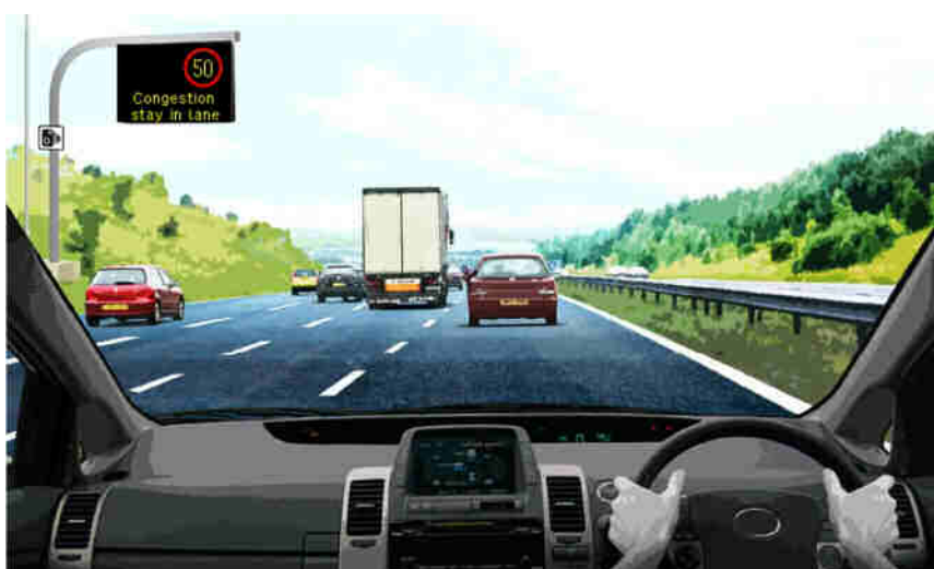
Figure 4D: Illustrative M1 J28 to J31 managed motorway scheme section operating with variable mandatory speed limits and information for road users.
