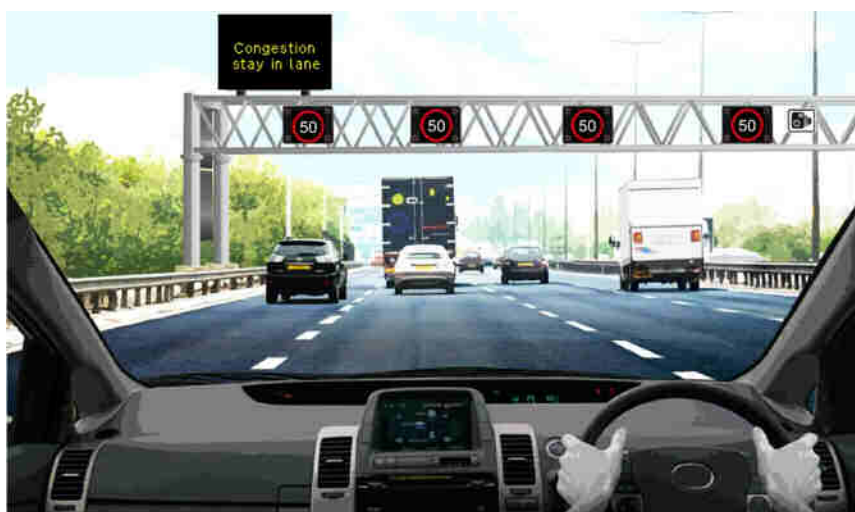
Figure 4C: Illustrative M1 J28 to J31 managed motorway scheme section operating with variable mandatory speed limits
