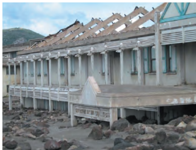
Figure 3: Government Headquarters submerged in ash and debris following the eruption of the Soufrière Hills volcano, Montserrat (Image courtesy of Dr. Sarah Petrie, DfID)
