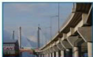
Golden Ears Bridge, Vancouver, B.C.
