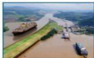
Panama Canal Expansion $5.3 B
