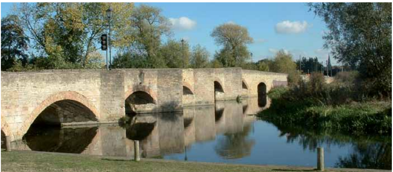
↑ River Nene, Thrapston Bridge
