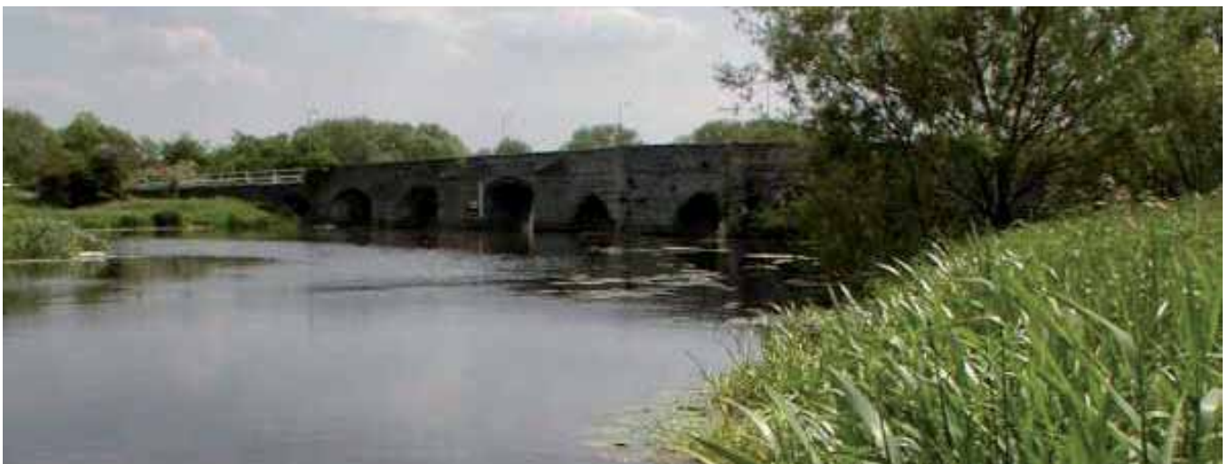
↑ River Nene, Old Road Bridge, Irthlingborough
