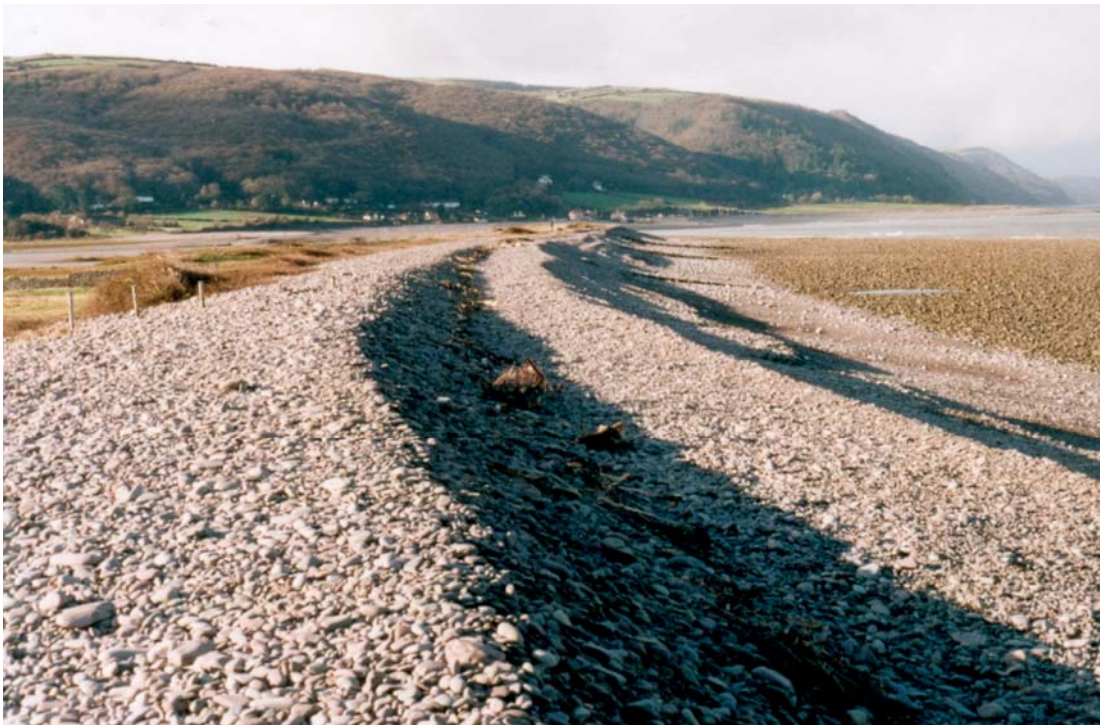
Figure 41. Barrier crest between E 14 and E15 viewed westwards on 14 th January 1999. The crest is relatively stable, and a secondary crest has accreted some 3-4m seaward of the original storm crest. Note the extensive low gradient boulder frame forming a dissipative lower foreshore. This feature imposes a depth limitation on the approach of very large waves, except for during high storm surge events.
