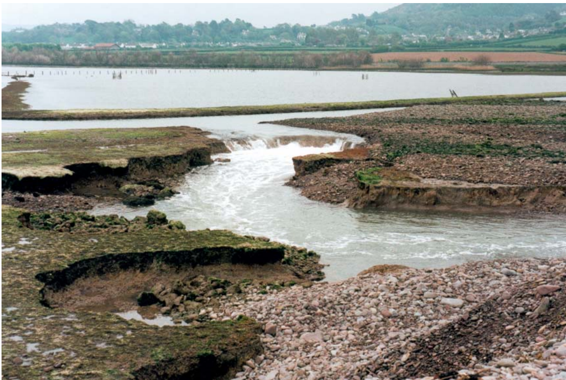
Figure 20. The NE arm of the breach channel on 5 th May 00. It has eroded rapidly headward since late 1998 and by Summer 2000 appeared to have assumed dominance over the southern arm which has evolved more slowly. Continued headward erosion would by July 01 result in linkage to the deep north-south trending drainage ditch that formerly directed flood waters towards the New Works sluice. Such linkage should result in more effective drainage of the lagoon altering its tidal regime.
