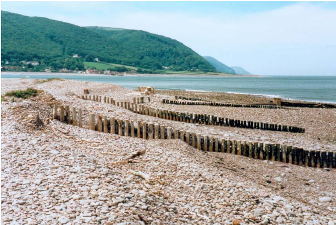
Figure 38. View west towards New Works from E08 on 19 th June 1998. The barrier is controlled by a series of timber pile groynes constructed in 1967-68 and which have promoted some beach accretion.
