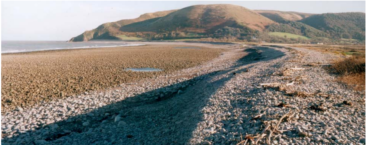
Figure 42. View east from E 13 over a stable portion of the barrier that has accreted at the crest (note the new berm deposited 1-2m seaward of the previous barrier crest). The wide low gradient boulder frame is seen comprising the lower foreshore and is effective at dissipating wave energy, perhaps contributing towards the stability of this portion.
