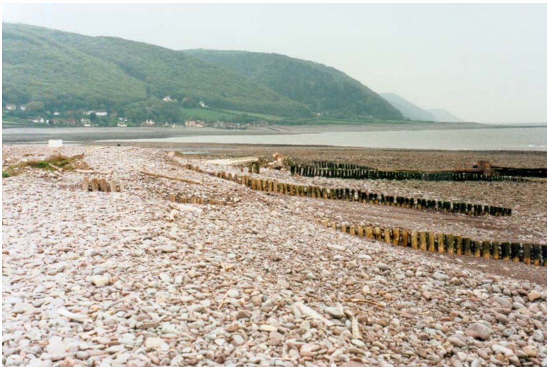
Figure 39. View west towards New Works from E08 on 4 th May 2000. Note that there has been accretion at the barrier crest and around the groynes in the foreground. However, foreshore lowering and crest recession is evident around the structures at New Works leading to their progressive destruction (compared with the June 98 situation). The barrier in this area is relatively low and is subject to overwashing although it has migrated much more quickly landward to the west of new works than here to the east.
