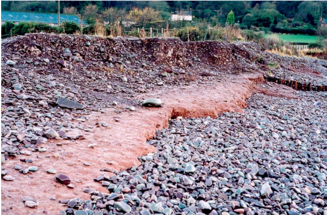
Figure 50. Depleted upper beach and eroded crest at Porlockford at the western extremity of Cell 3, 8 th Dec-00.
