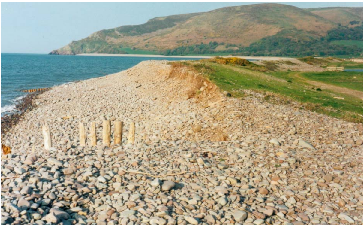
Figure 14. Erosion cutting into the crest of the “stable” barrier at Profile E09 on 4 th May 2000. Note the vegetated backslope in the foreground and a less well vegetated section in the mid-distance close to the war memorial. Such areas indicate parts of the barrier that are becoming increasingly subject to seepage and occasional overwashing. The disturbance produced is such that a continuous vegetation cover cannot become established.
