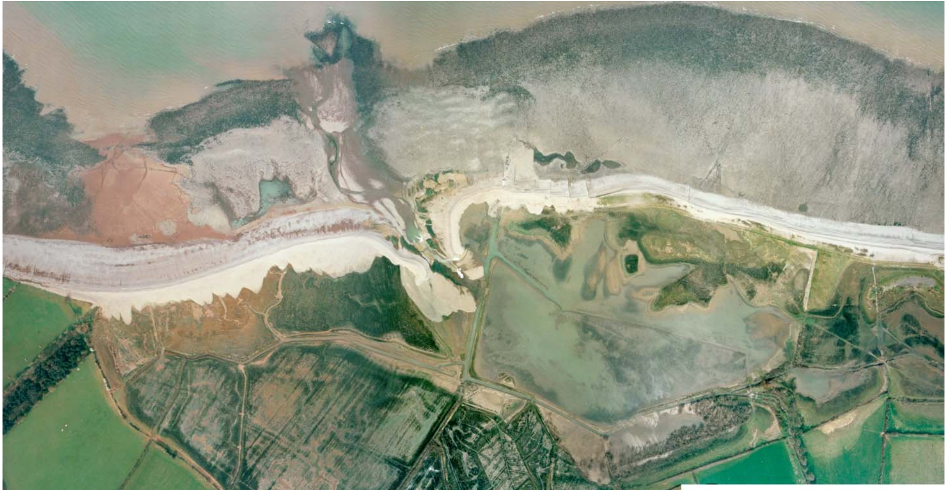
Figure 6 Vertical aerial photograph mosaic of the breach and lagoon at 1216hrs on 1 st April 1999. Note that the photos are non-rectified and should not be used for direct measurement of features.
