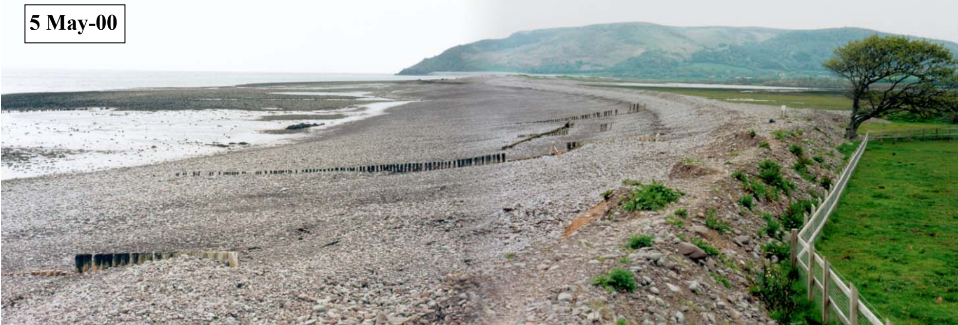
Figure 22 Views eastwards from Porlockford Cliffs showing the western extremity of the barrier. Note the timber pile groynes – nos. 4 (foreground), 5, 5a and 6 - that have been deliberately lowered in places to permit eastward drift. The May-00 beach appears to have accreted around groynes 4 and 5, but has suffered losses around groynes 5a and 6 by comparison with Jun-98. The crest also appears to have retreated by several metres. This area was one of the most vulnerable in the 1980s when significant “breaches” occurred on an annual basis. Since 1998, this area has suffered overwashing rather than serious breaching. Crest flattening is followed by natural rebuilding a short distance inland. Overall, the barrier is lower, flatter and wider than its 1980s counterpart and is potentially a more effective dissipater of wave energy.
