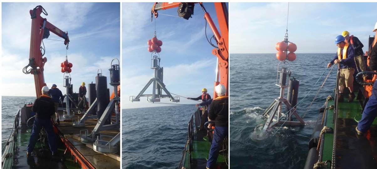
Figure 8. Left, lander being picked up from the deck of MTS Grey Bear using hiab winch, wire and the IXSEX 2500. Mid, lander being steadied and swung outboard. Right, lander being lowered into the water before final positioning and lowering to seabed.
