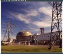
Windscale is part of the Sellafield site in Cumbria. The site area is 14 hectares. It comprises three reactors, two of which were shut down in 1957. The third was closed in 1981. A fire damaged one of these reactors (Pile 1) in 1957, making its decommissioning a significant challenge.
