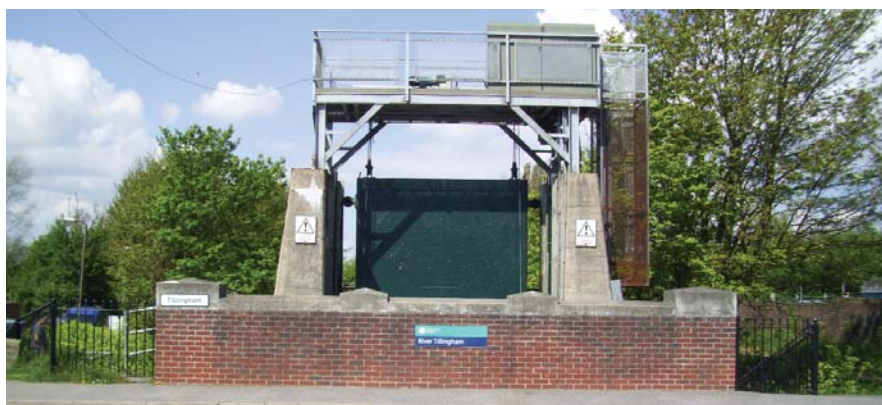
↑ Sluice Gate on the River Tillingham, Rye.
