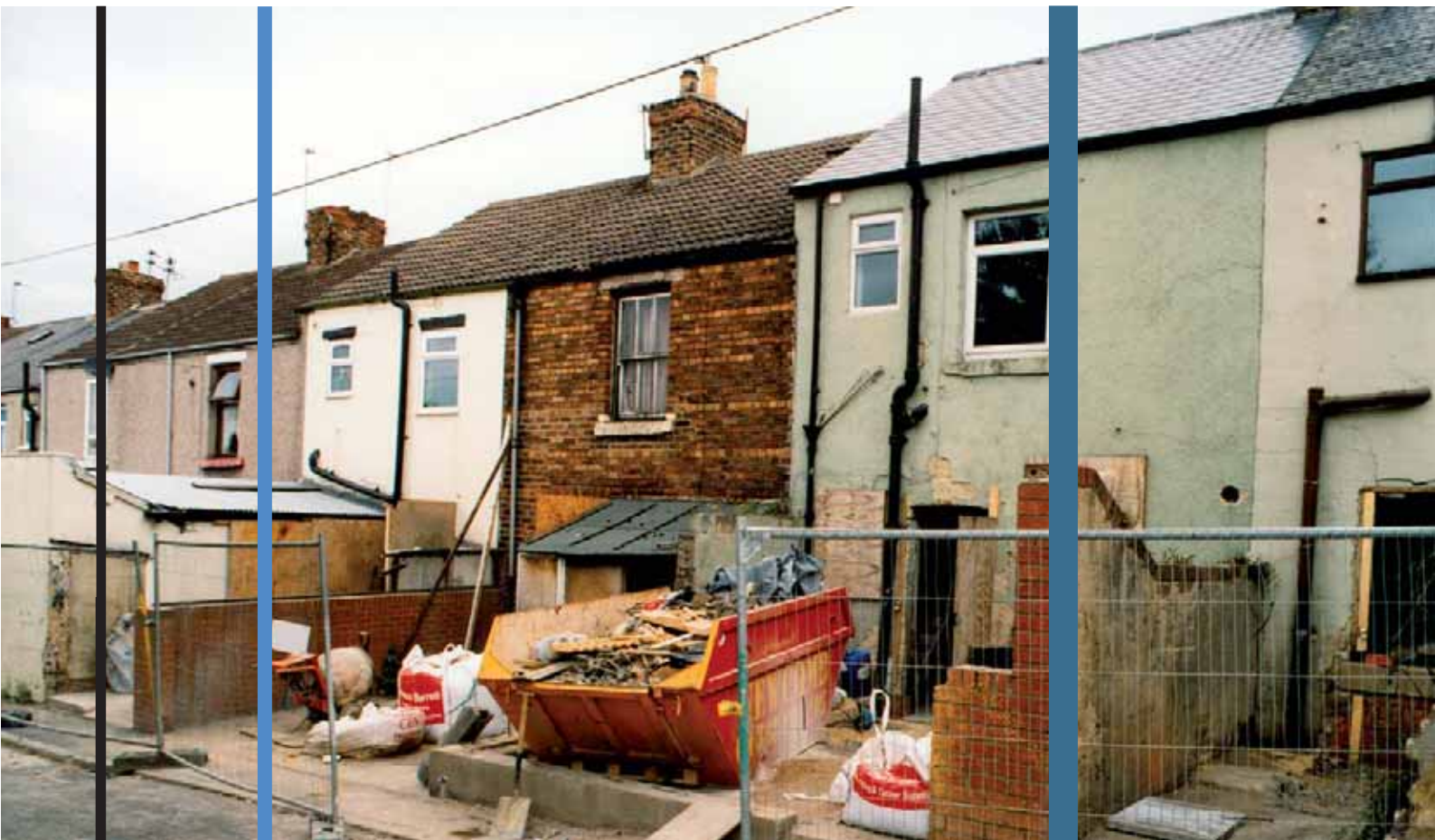
Subsidence repair work in the North East.
