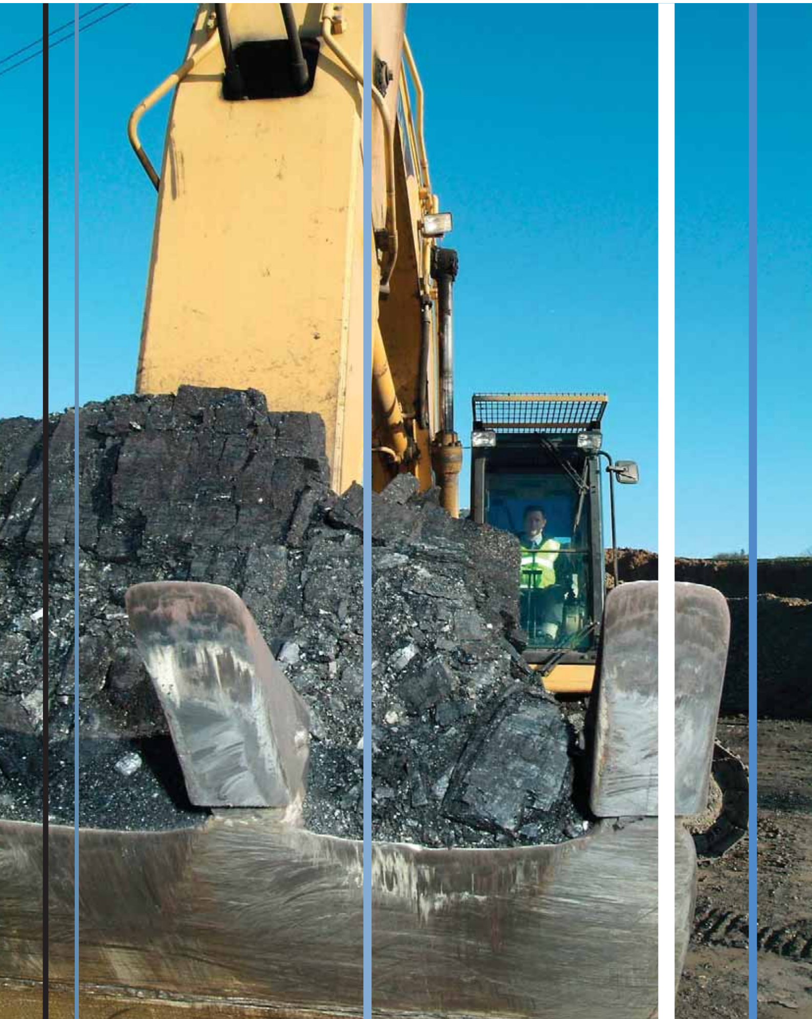
UK Coal's Stoney Heap surface mine.
