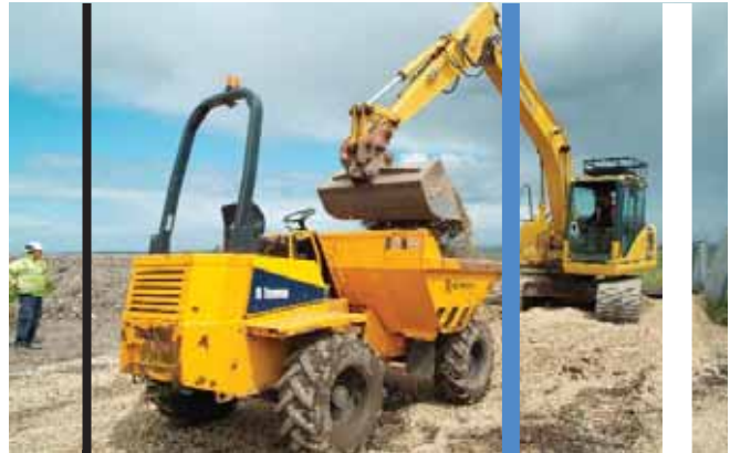
Dawdon minewater treatment scheme under construction.
