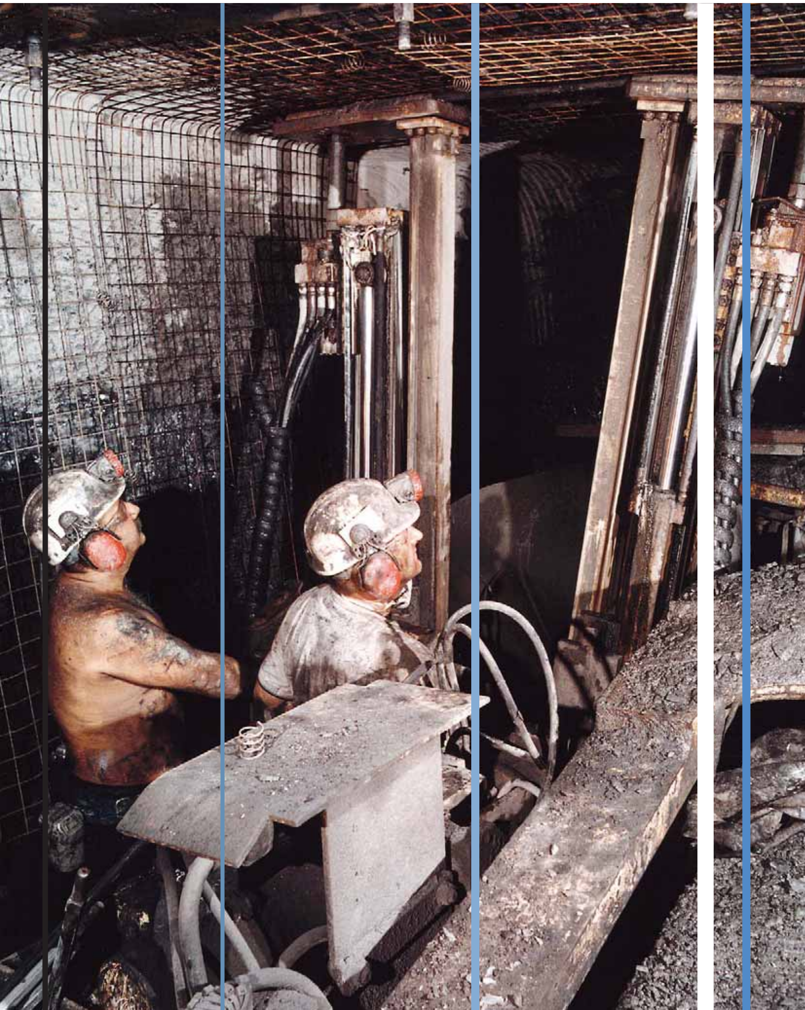
Roofbolting at Maltby Colliery.
