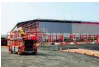
Construction of the Royal Mail Depot, Northampton
