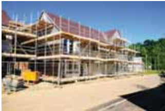
Construction at Westlake, Northampton
