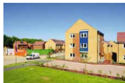
Construction at Billing Lane, Northampton
