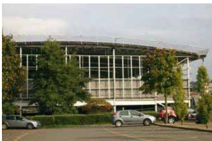
Construction of Abbey Retail Park, Daventry
