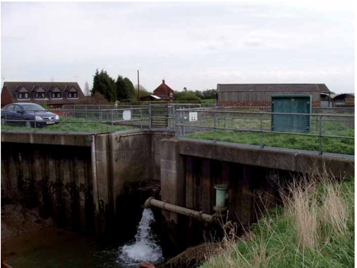
↑ Barrow Haven Sluice
