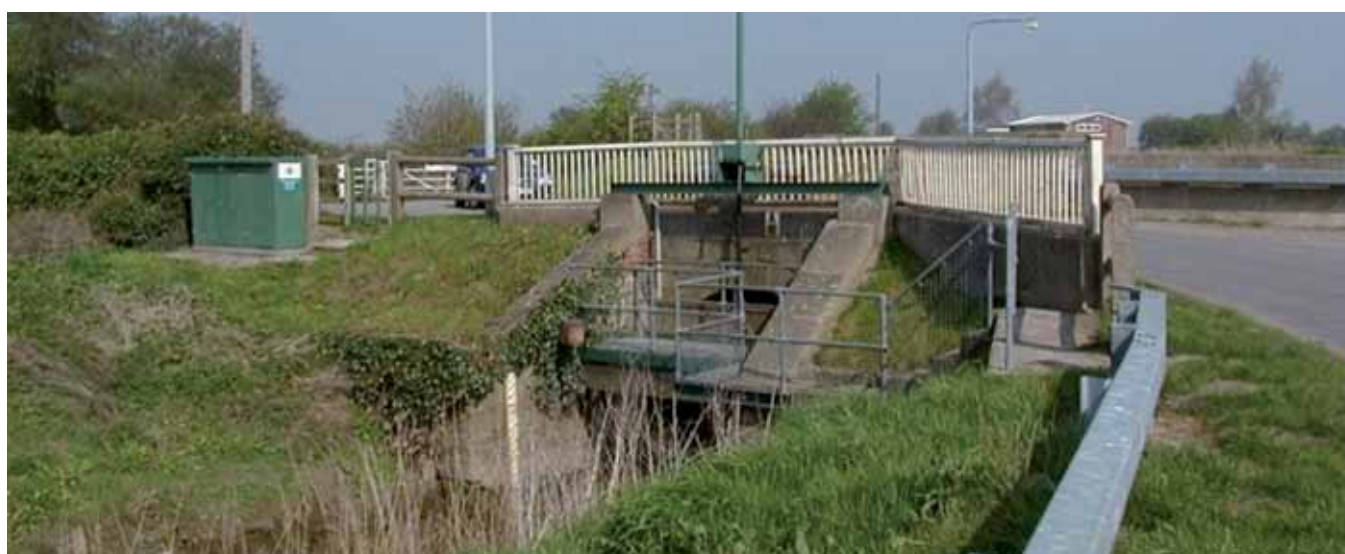
↑ Winterton Beck Outfall
