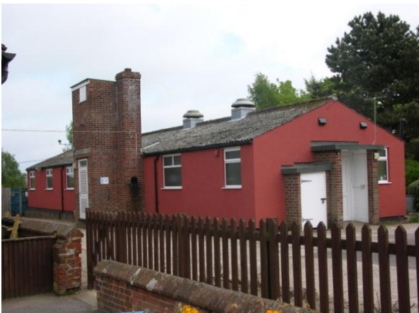
Figure 7 Reepham primary school canteen after the external insulation had been installed
