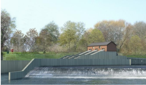
Figure 2: Visualization of the Archimedes screw turbine at the Shrewsbury weir site
